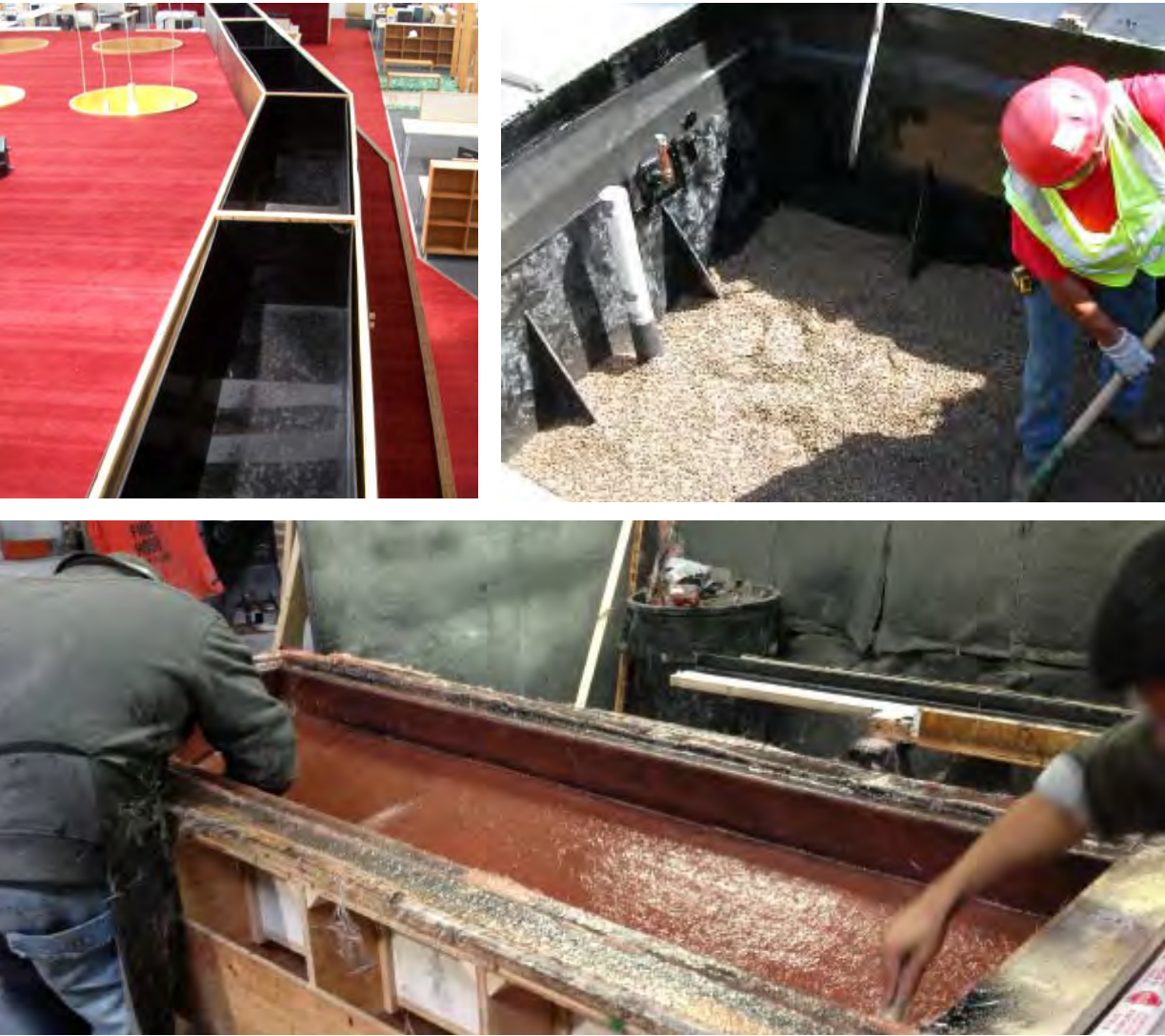
ABOVE, TOP Installations showing use of welded planter liners in the field, large and small.
